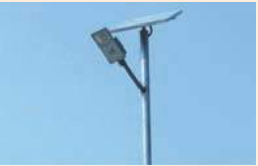
Installation of Solar Street Lights
