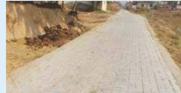
Interlocking Pavers and Drains 1
